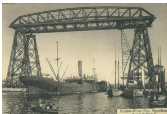
Fig. 19, Puente Avellaneda, Tarjeta postal, c.1919
